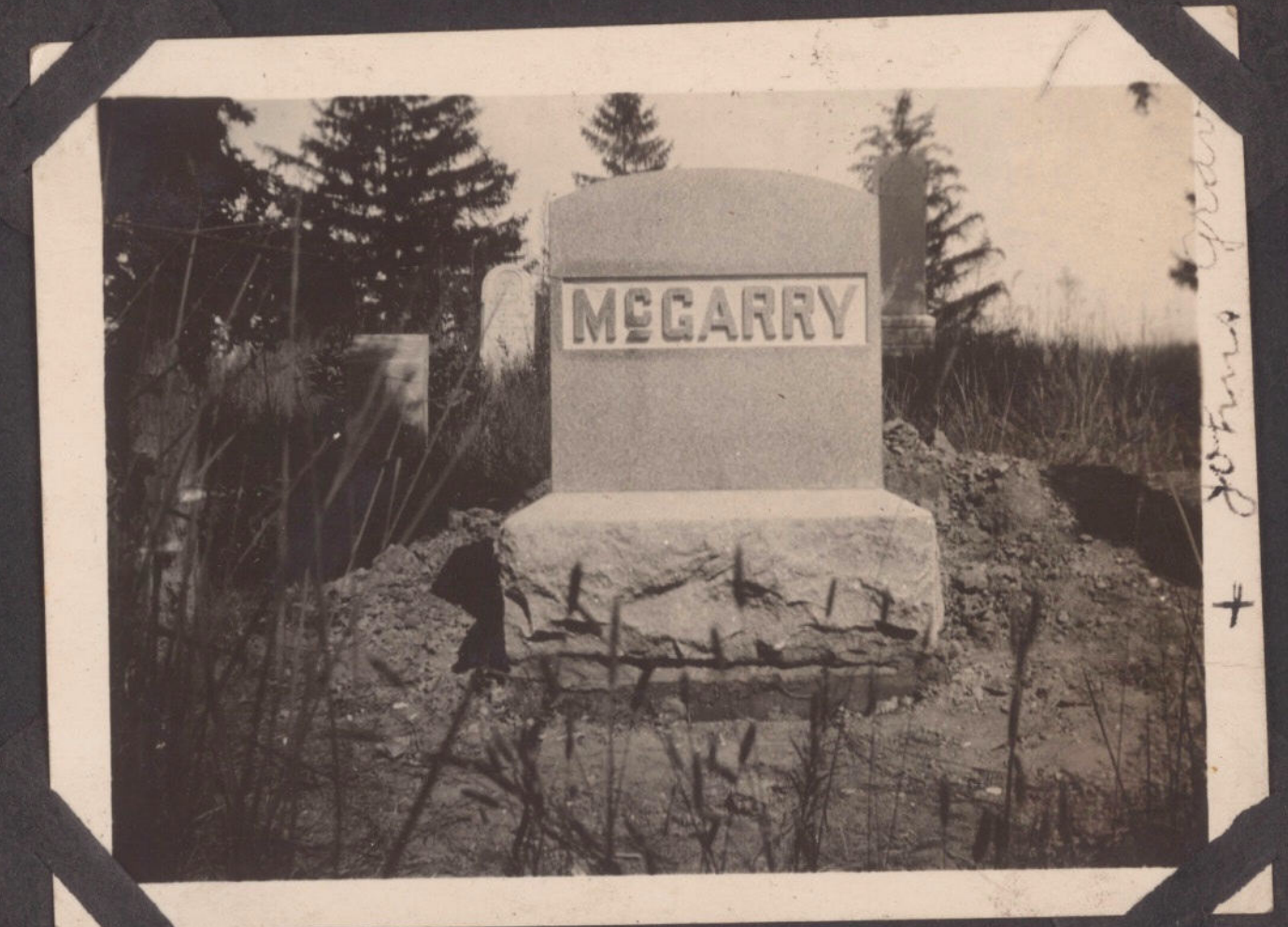
Grace took these the day we put the monument up before we hauled the dirt away from the foundations for monument and marker. Thier markers are alike - uncle John McGarry.
